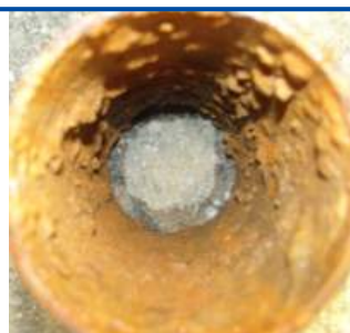
1st inspection (January 29, 2008)
