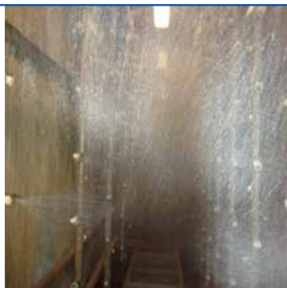
100% spray with hardly any clogged nozzles
