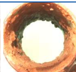
3rd inspection (May 6, 2009)
