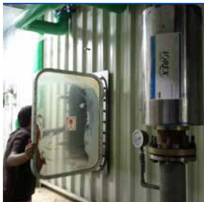
Air handling unit with IOREX (100A)
