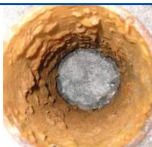
2nd inspection (July 25, 2008)
