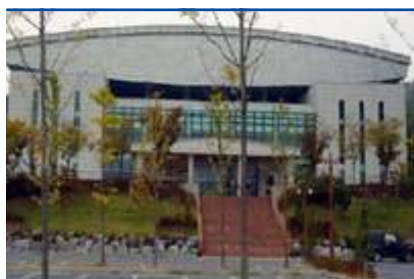
Gyeonggi-do pyeongtaek-si Leechoong Cultural and sports centre _ IOR-80A
