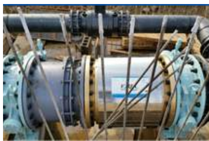
Saemangeum Industrial Complex Development Project _ IOR-600A
