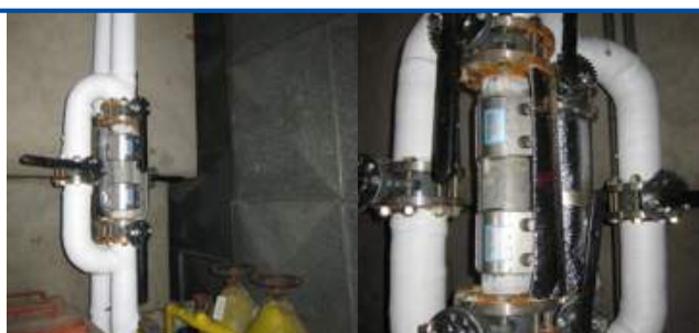
Installation of the inspection point
