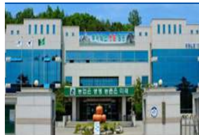
Gyeongsangbuk-do Technical Center for Agricultural Cooperative _ IOR-80A
